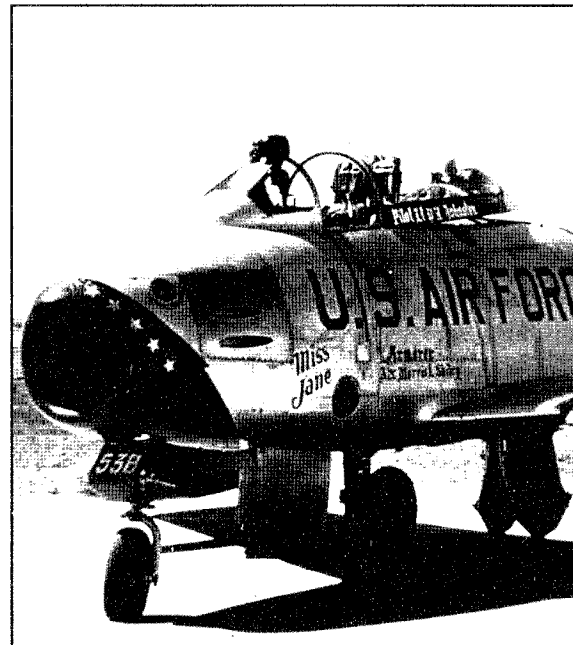
"Miss Jane" was the F-86F flown by Lt. Don Johnson when his squadron was based at Kimpo AB, Korea in 1957. Note that the Sabre is equipped with the latest wing configuration - extended wingtips, 6-3 leading edge and slats. (credit-Don Johnson)
